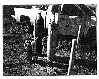
Exhibit 3. Nitrogen delivery system for the SDC-9<sup>TM</sup> bacteria injections
