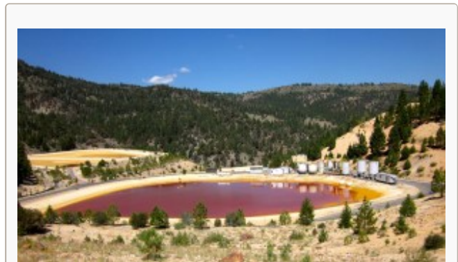
Leviathan holding ponds and treatment system used by the water board at the site. Photo/Lahontan Water Board
