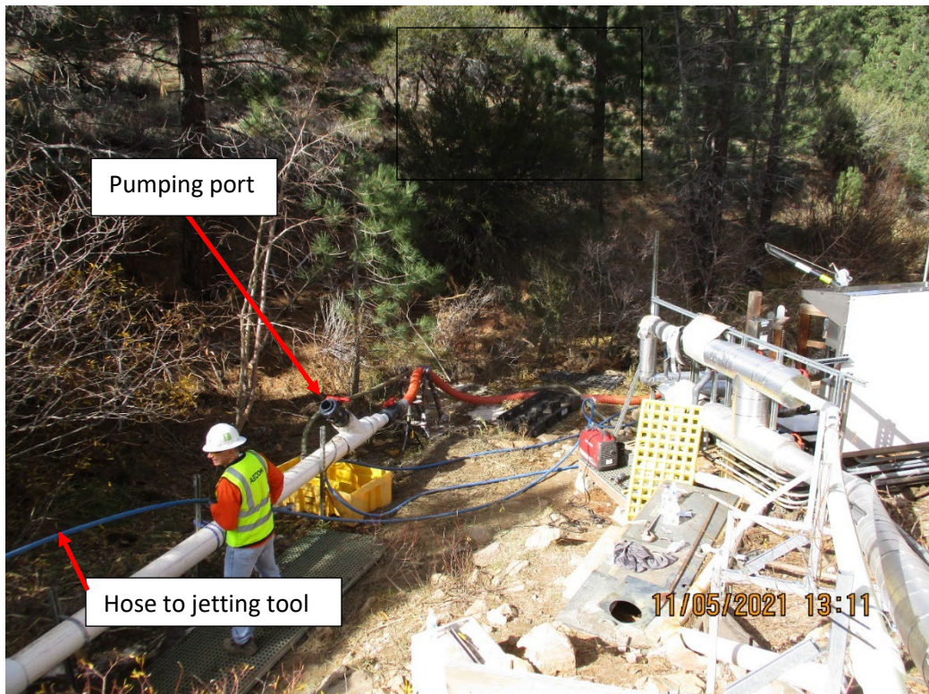
Photo 10 – November 5, 2021, Jetting and pumping activities at the CUD
