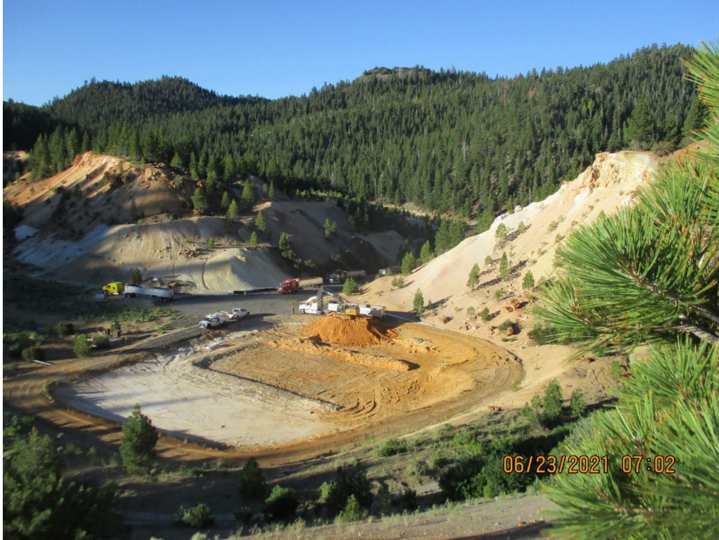
Photo 1 – June 23, 2021, Sludge stockpile and disposal activities at the pit clarifier
