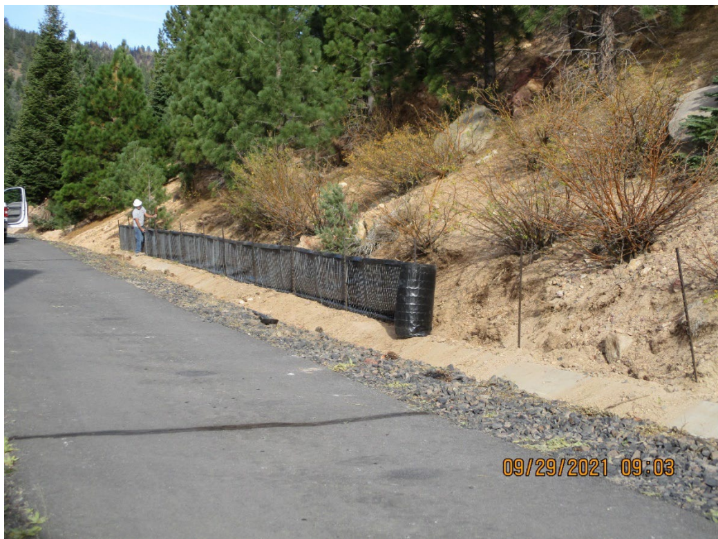
Photo 4 – September 29, 2021, Installation of new reinforced silt fence near Pond 1
