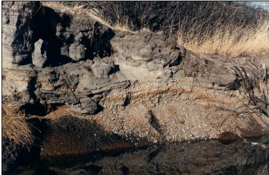
Figure 13. Examples of stream bank failure along Squaw Creek in Squaw Meadows. Stratigraphy exposed in alluvial stream bank shows fine-grained fluvial and lacustrine sediments overlying less resistant sand and gravel layers.
