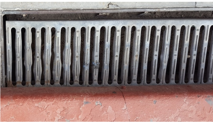
Photo No. 1 Sierra Boat Company: Hydrographic Area B, accumulated sediment and dirt in trench drain that leads directly to pre-treatment vault.
