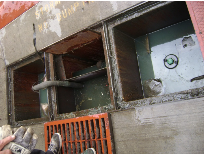
Photo No. 3 Sierra Boat Company: Hydrographic Area B, pre-treatment vault filled with water from boat washing activities.
