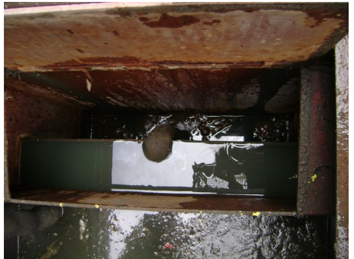
Photo No. 4 Sierra Boat Company: Hydrographic Area B, pre-treatment vault with sludge adjacent to the outlet to surface waters.
