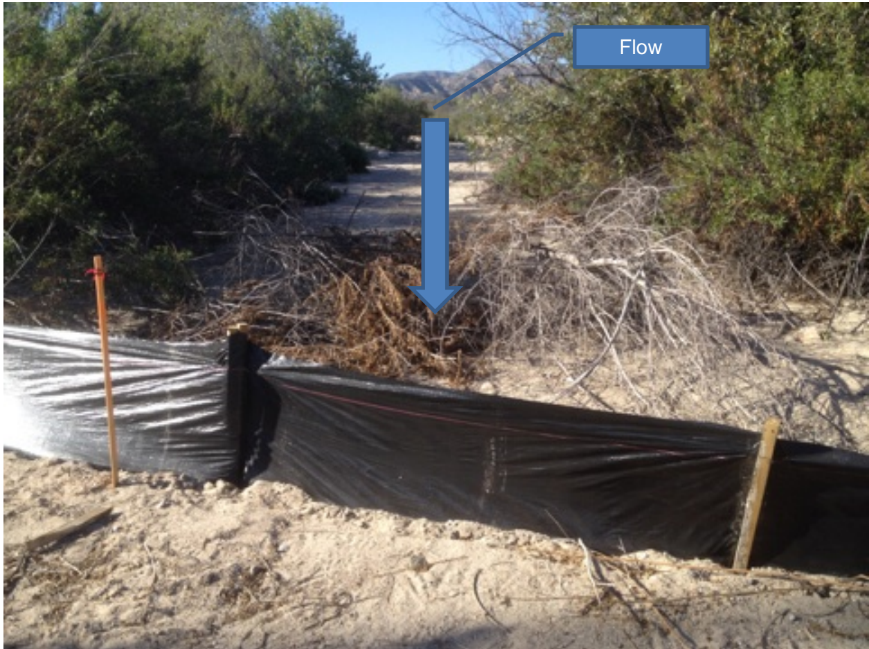
Picture 13: View North of silt fence installed across Cajon Creek Channel.
