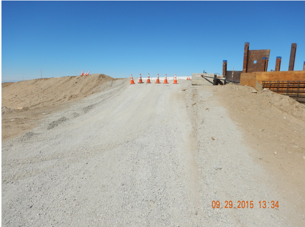
Picture 31: View facing north along construction access road (west of Sheep Creek) to active paving activity along the SR 138 alignment.
