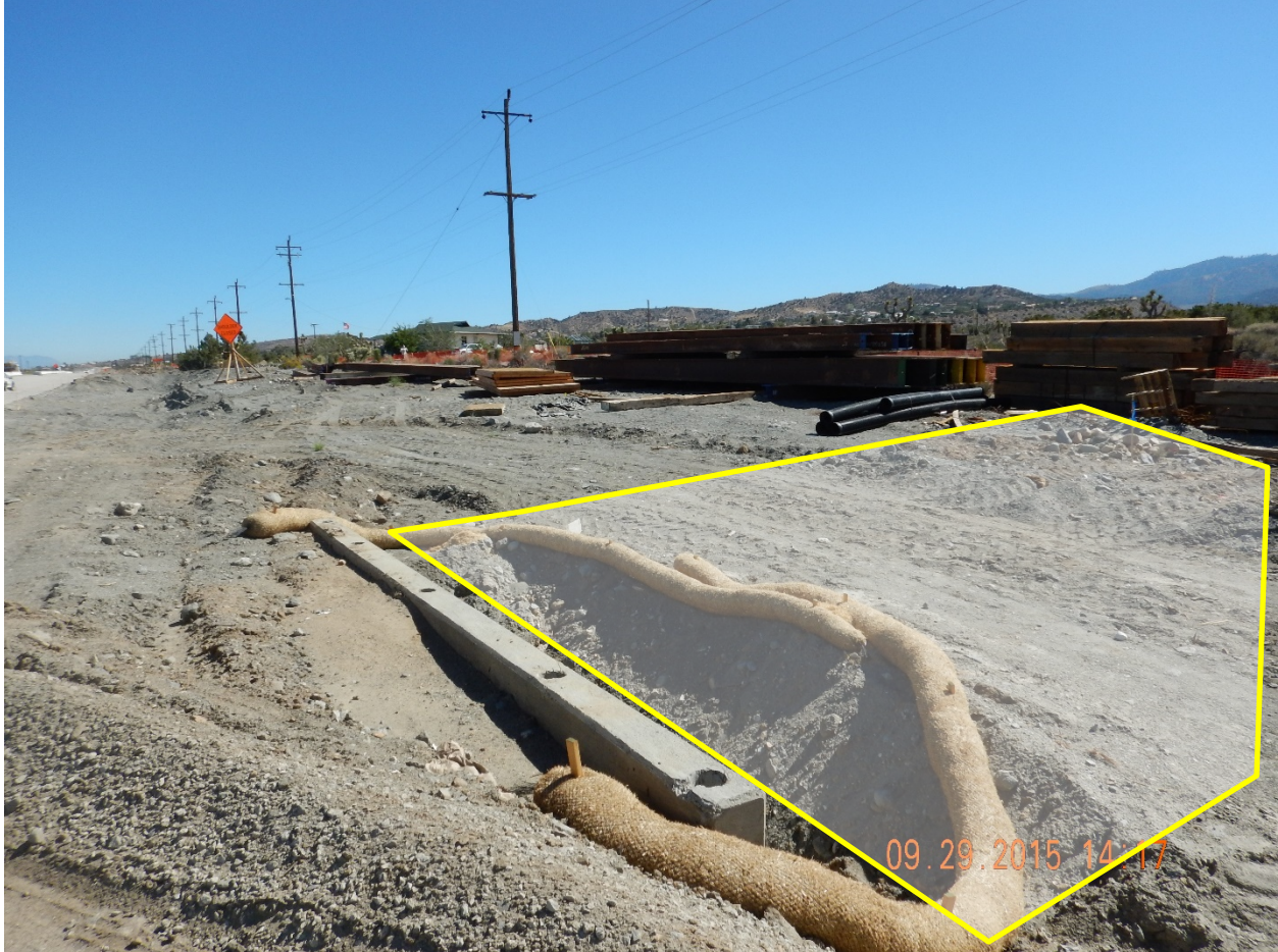
Picture 4: View South East of unpermitted temporary impact at Drainage ID 54. Note fill from access road in the stream channel (rough outline of area in yellow).
