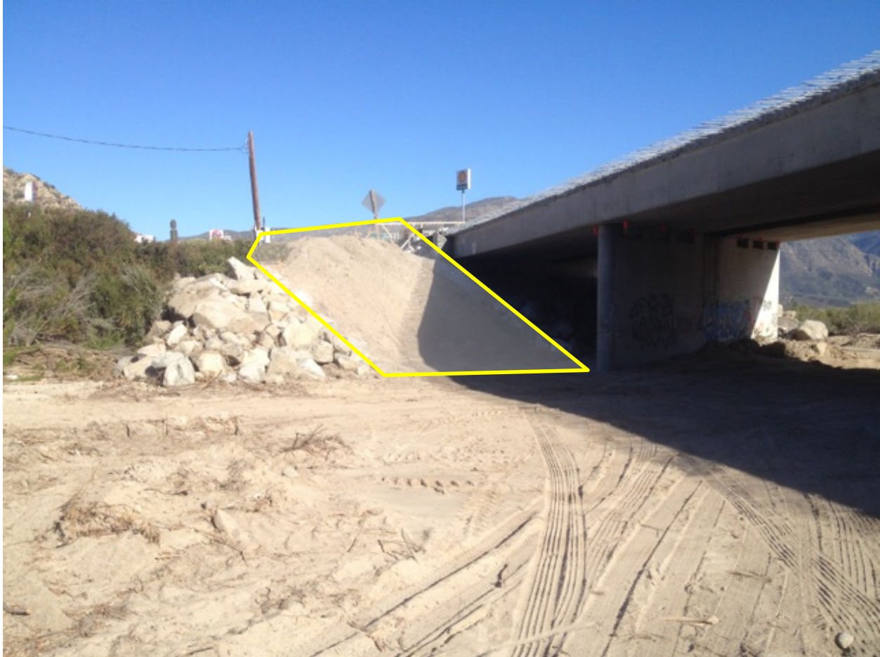
Picture 10: View East of Cajon Creek North East bank. Note the absence of erosion and sediment controls on the exposed bank (rough outline of area in yellow).
