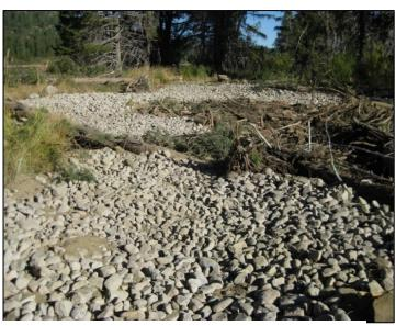
Photo 2 – Sand bag berm removal and content stabilization conducted in September 2018, as part of the 2018 implementation and Monitoring Plan.
