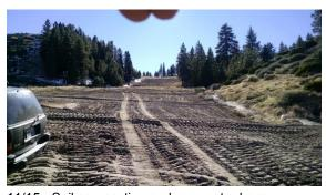
11/15 - Soil compaction and new water bars on "Mambo" slope; seeding is planned to be done before opening of their season
