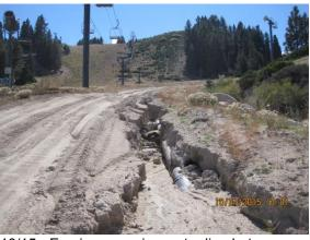
10/15 - Erosion exposing water line between a reservoir and storage tank for snow making
