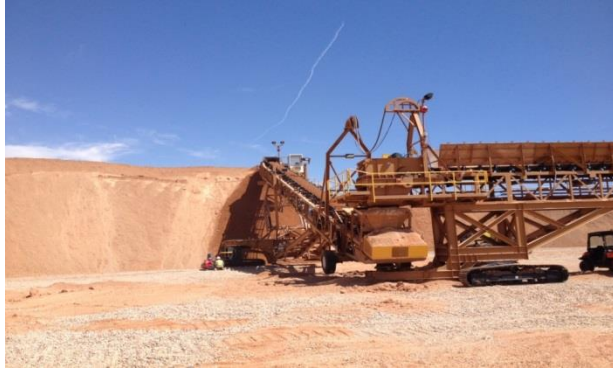
Figure 5: Cyanide solution conveyance piping. The black pipe conveys metal-bearing solution from the leach pad to the Plant, and the brown pipe conveys barren solution from the Plant back to the heap.
