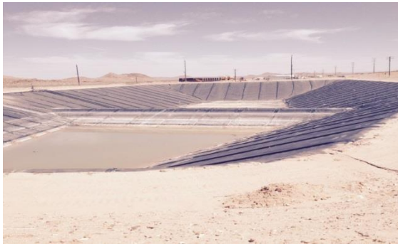
Figure 3: Surface Impoundment holding storm water run-off from the heap leach pad and groundwater used as "make-up" water for the cyanide solution.
