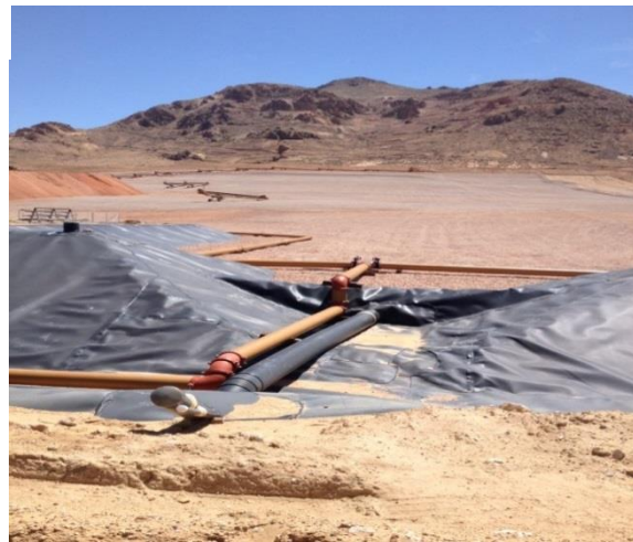
Figure 4: Close-up of heap leach pad being loaded with ore.
