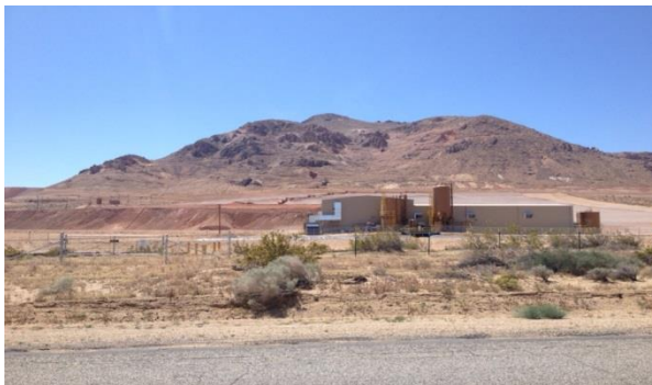
Figure 2: Soledad Mountain in background; Merrill-Crowe Plant in foreground; heap leach pad with ore to the left of the plant, and ready for ore behind and to the right of the plant
