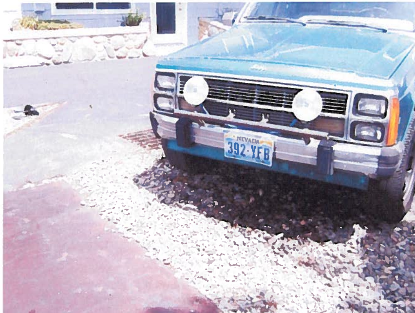
Photo 15. Truck dripping antifreeze onto drain rock along bulkhead, between maintenance and office buildings.
