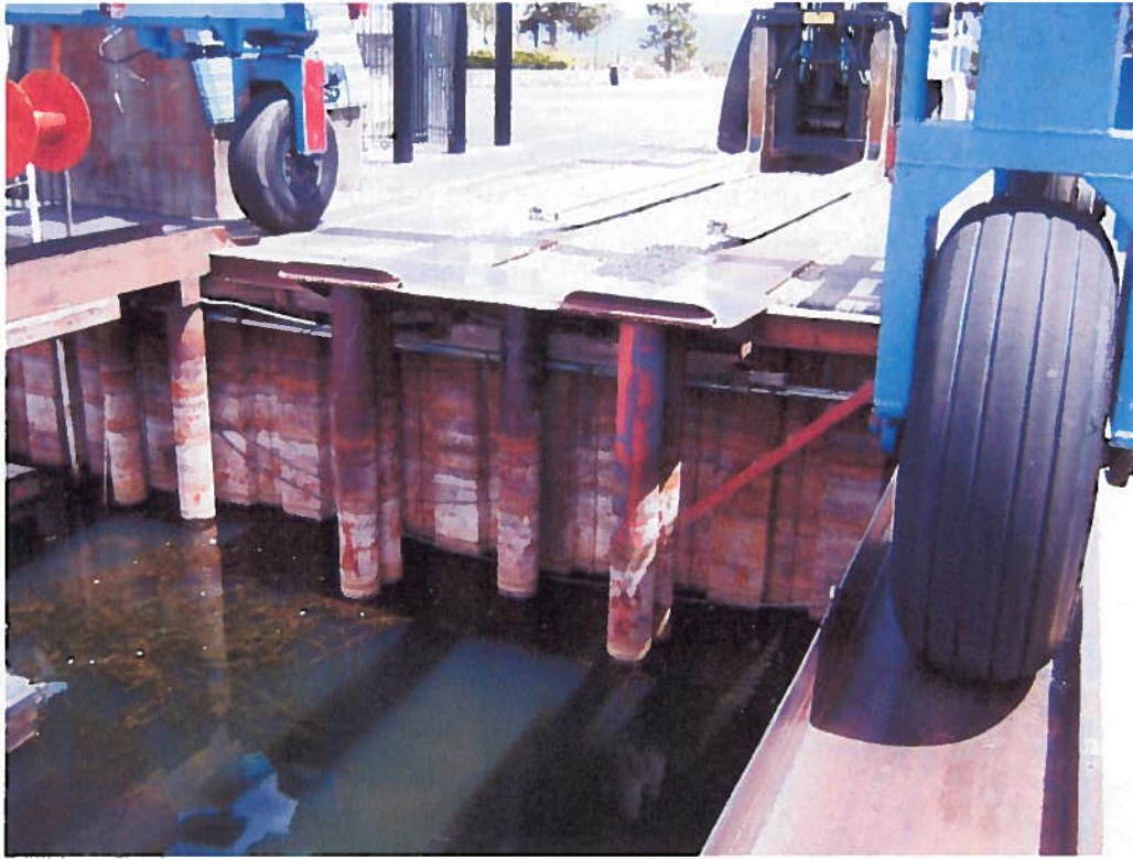
Photo 19. Bulk head of boat lift, facing east.
