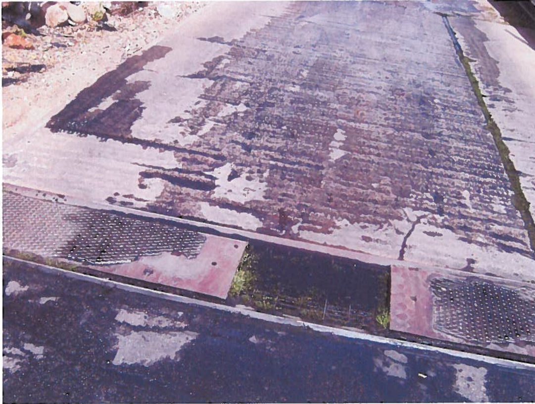
Photo 11. Clogged slotted drain along boat ramp, located on northeast side of the marina, along the west side of the ramp facing the Lake.
