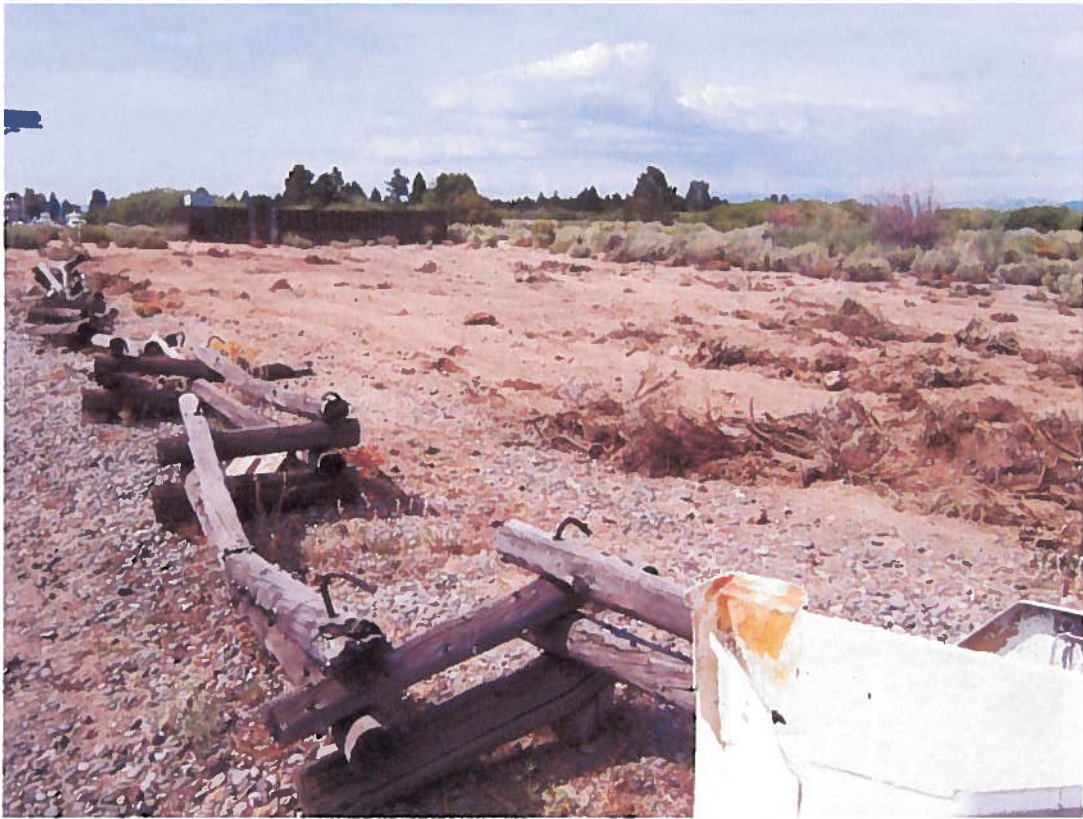
Photo No. 2. Looking east northeast at graded area.
