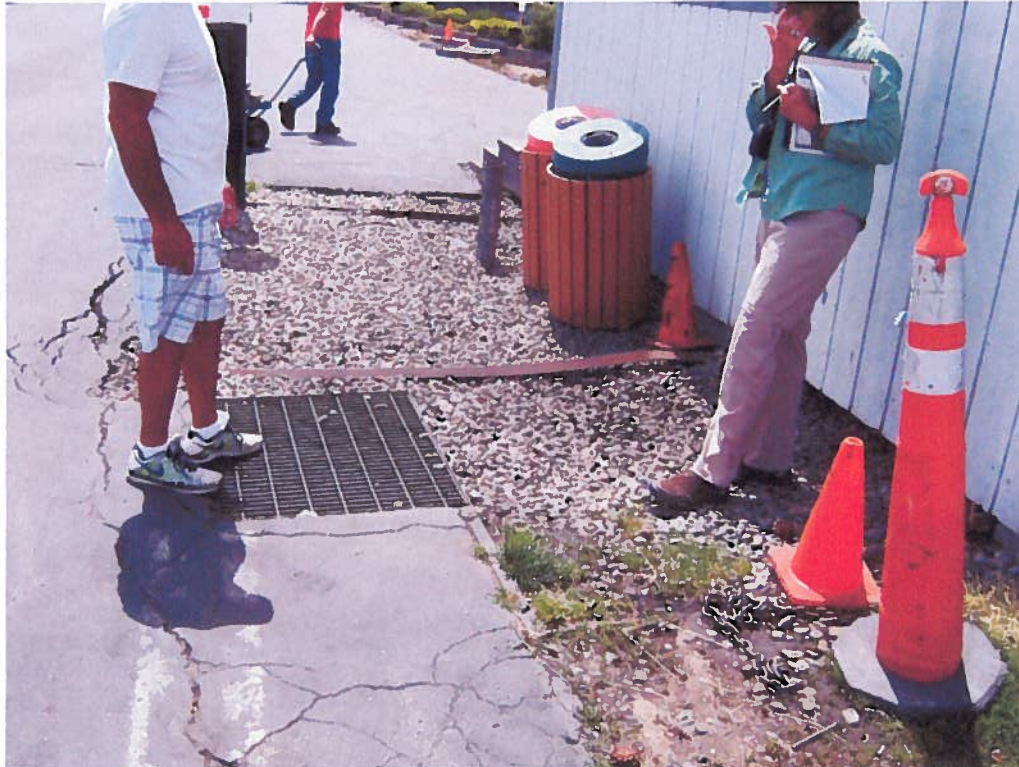
Photo 16. Drain area on southeast side of Maintenance Building, facing in a southwest direction. Mr. Spinnato is on the left, Tobi Tyler is on the right. New drain rock had been installed where the area had previously been excavated to determine why this area had been clogging.
