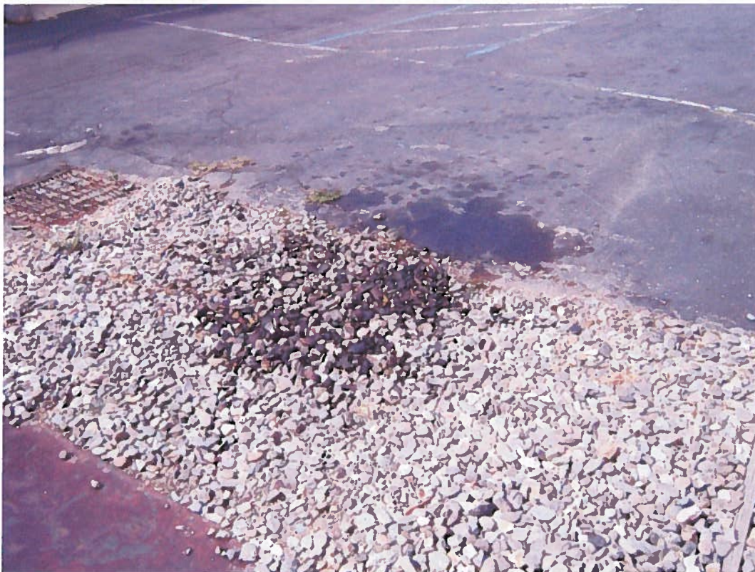
Photo No. 9. Antifreeze-stained gravel in drain rock on northwest corner of maintenance building. Looking east northeast, marina bulkhead is immediately behind me.
