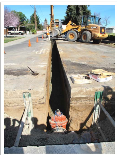
Photo 1 Construction takes place to connect the communities to Yuba City.
