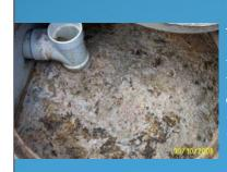
Proper schedule 40 PVC Inlet T ½ to 2/3 the depth of the tank (picture at right) prevents back-ups into FSE, and does not allow the influent wastewater to push the FOG layer down and allow shortcircuiting.
