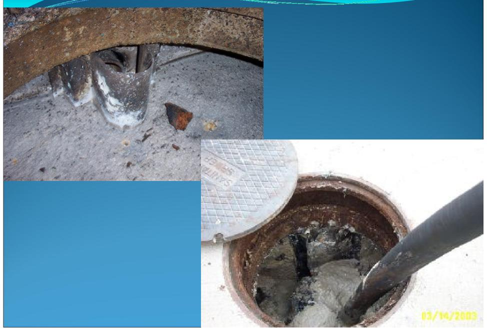
Flexible material (SD-35 plastic) attached to wall in interceptor will eventually be floating in interceptor
