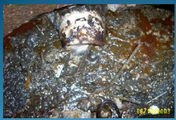
No inlet T (picture at left), allowing FOG buildup in front of discharge pipe.
