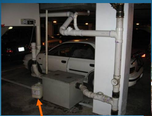
Trap in basement with additives (enzymes) added before trap. Heavy FOG in downstream sewer line.
