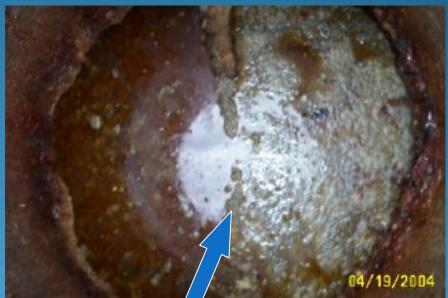
Baffle irregular, deteriorating
