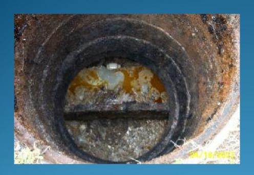
Outlet Ts can be too short, allowing shortcircuiting. Some rely on baffle in front of outlet pipe but this is not efficient for FOG control
