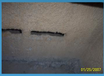
Mid-wall Baffle (or 2/3 baffle wall)- deterioration. Will probably need interceptor certification to confirm deterioration or leaks (gravel in bottom of tank in many cases is indicator)
