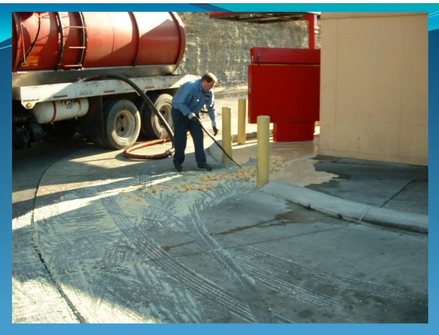
Automated grease recycle container overflow due to faulty level indicators
