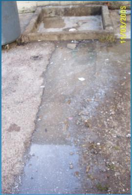
Uncovered Mop Sinks cause I/I to sewer system and many times the mob sinks are upstream of the grease interceptor. Outdoor mop sinks should be covered.
