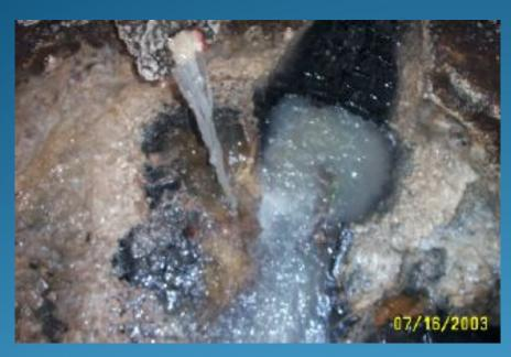
Identify FOG impact in sewer line. Note: Major impact may be 2 or 3 manholes downstream of FSE due to cooling of FOG
