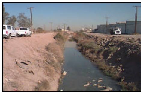
Figure 192 - Tula West Drain downstream of Hidrogenadora Nacional (Jan 1998)
