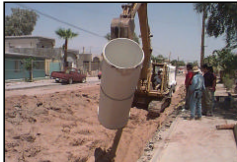
Figure 214 - South Collector repairs underway (Jul 1998)
