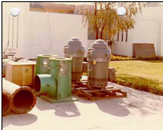
Figure 47: Equipment awaiting installation at Pumping Plant No. 1 (Mar 1982)
