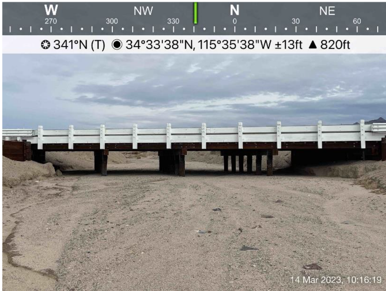
Photo 2: Upstream View of Lanzit Ditch Bridge, Facing North
