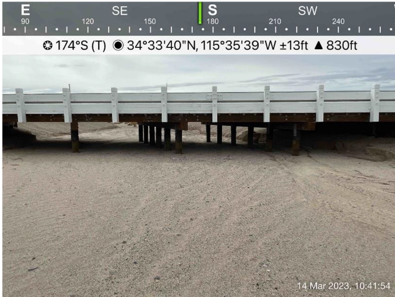
Photo 1: Downstream View of Lanzit Ditch Bridge, Facing South
