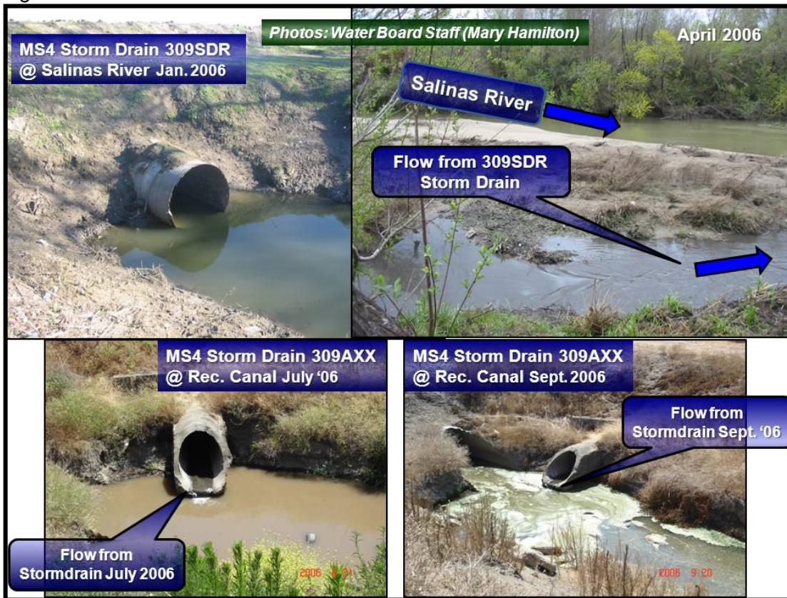
Figure 3-39. Photo documentation of MS4 storm drain outfalls.
