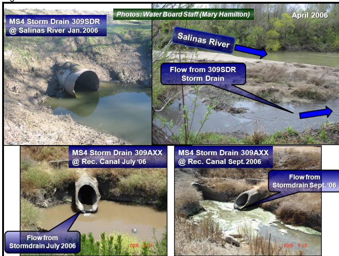
Figure 3-39. Photo documentation of MS4 storm drain outfalls.
