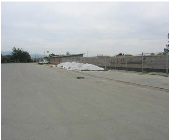
Photo 3. Salinas Sports Complex Municipal Stadium
