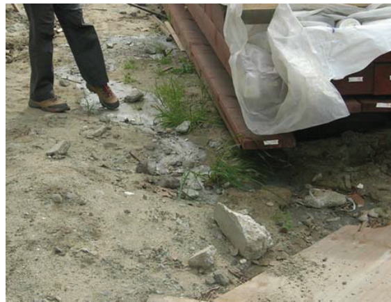
Photo 4. Freight Building Rehabilitation project
