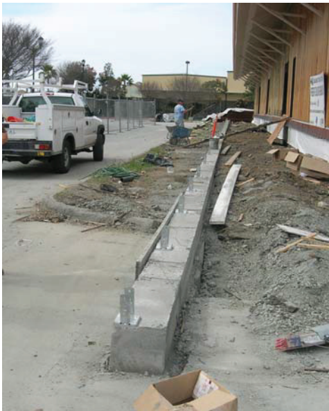
Photo 5. Freight Building Rehabilitation project
