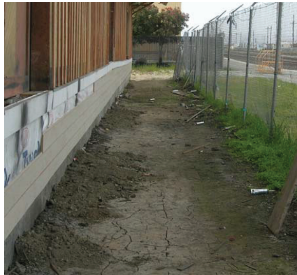
Photo 6. Freight Building Rehabilitation project
