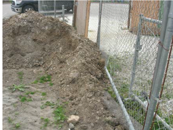
Photo 2. Salinas Sports Complex Municipal Stadium
