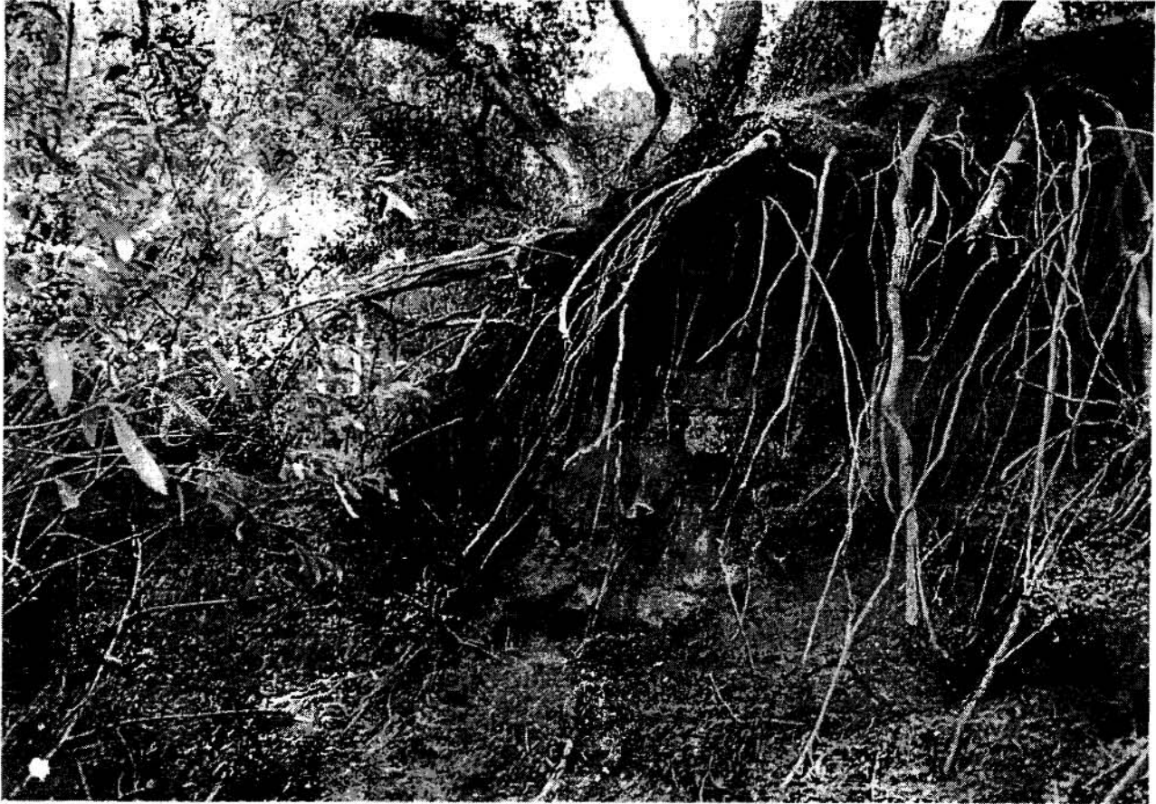
Figure 20. Bank Collapse on West Bank of Waddle Island
