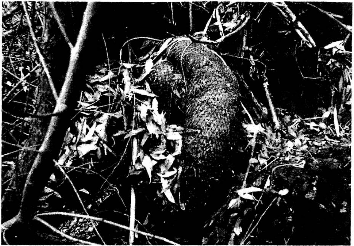
Figure 4. Biolog Binding Debris Jam
