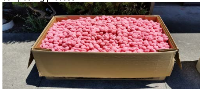
Fuzzy Filters at Graton WWTP
