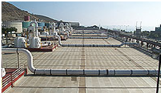
Point Loma WWTP
