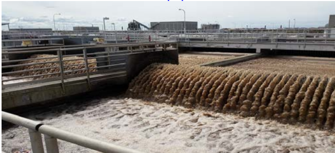
City of Roseville WWTP
