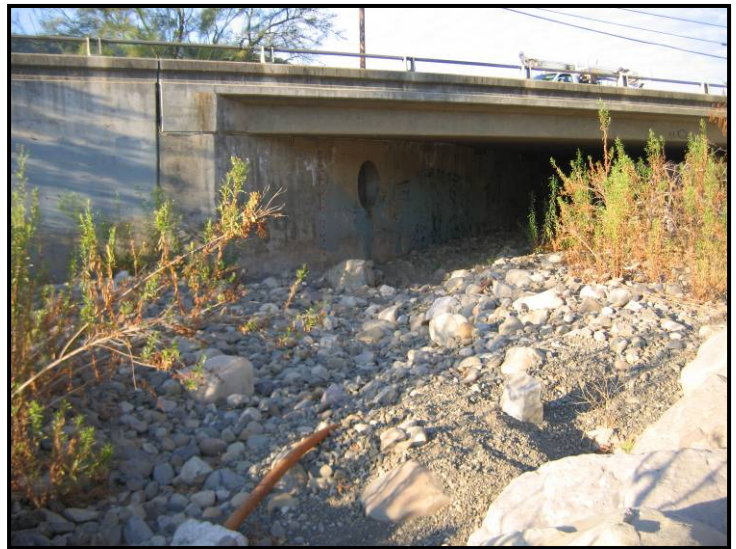
View downstream from site looking towards Ojai Ave. bridge
