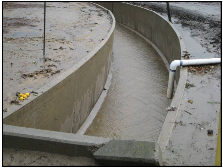
View upstream (NE) from sampling location
