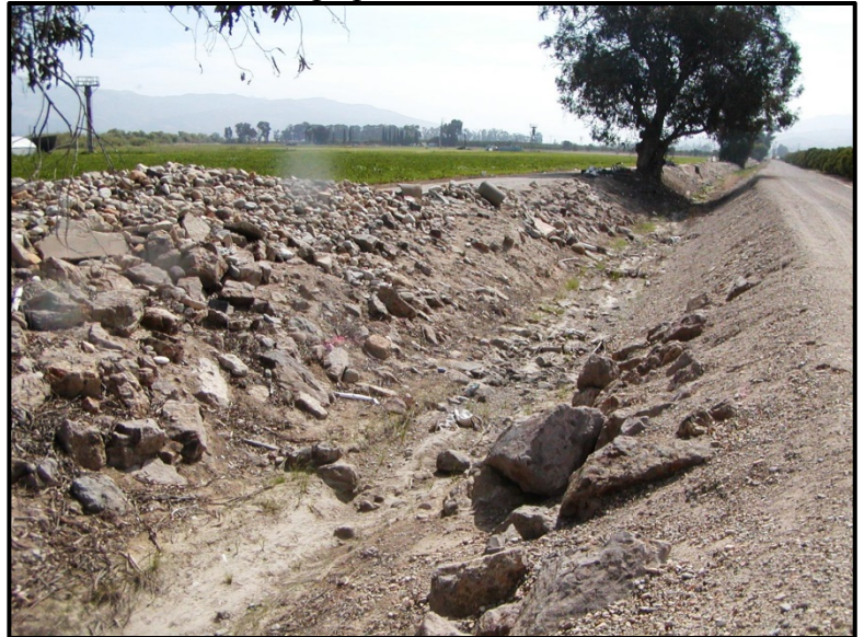
View of site looking upstream
