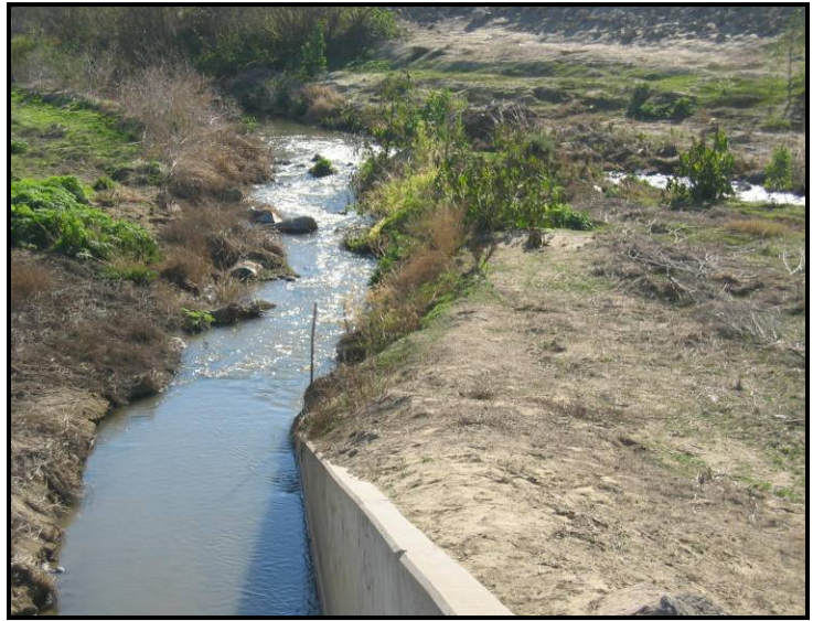
View toward SW looking downstream an ag drain before the confluence with Revolon
