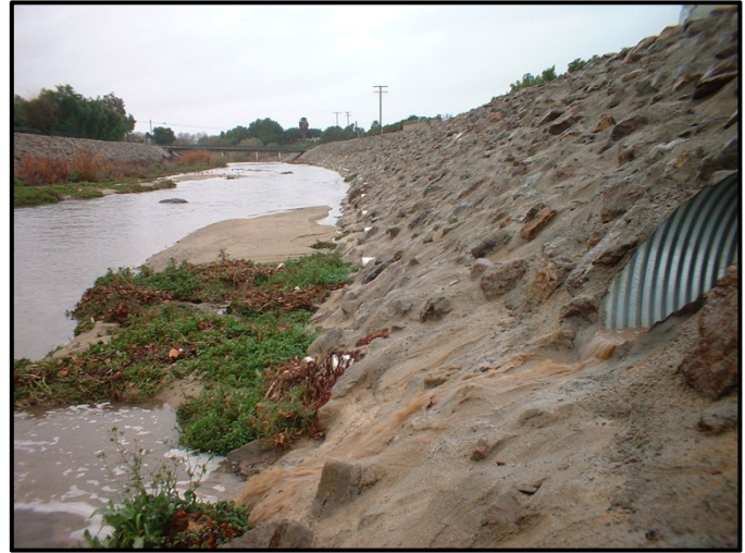
View of pipe discharging into Arroyo Simi
