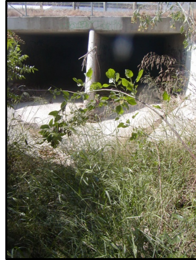
View of site (S) toward Hwy 126
