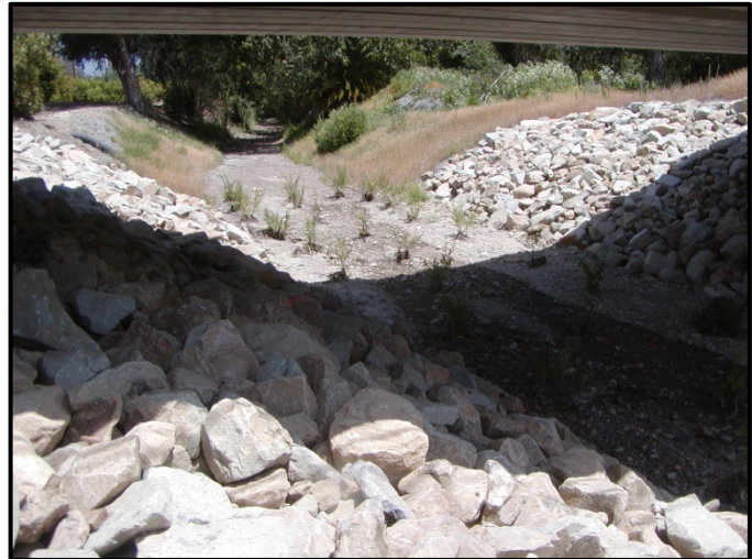
View upstream at the bridge
