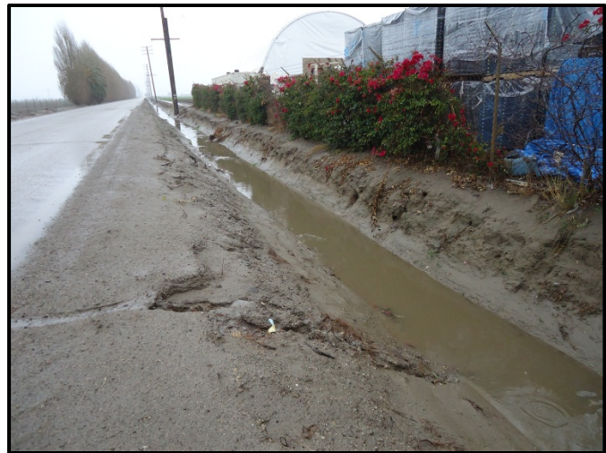
View at site looking upstream
