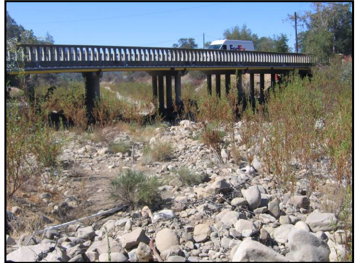
View downstream at the Grand Ave. bridge
