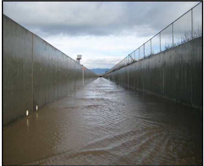
View upstream (NW) facing gage #781
