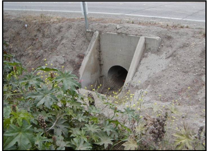
View toward SE of culvert draining runoff from CSUCI campus.
