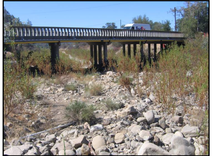
View downstream at the Grand Ave. bridge
