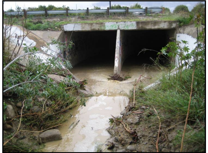
View of site (S) toward Hwy 126 bridge
