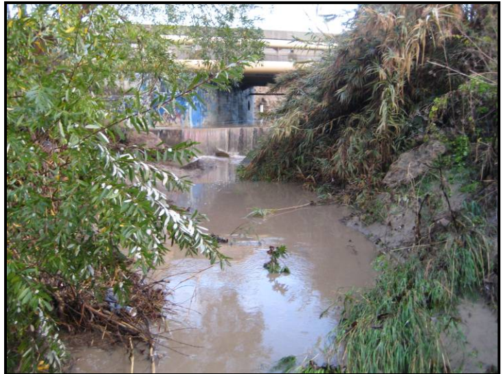
View upstream (N) from sampling location toward Hwy 118 Bridge
