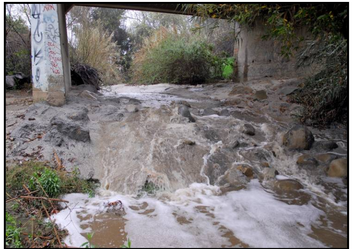
View upstream at the bridge pier
