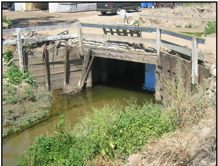
View toward the NE (looking downstream)
