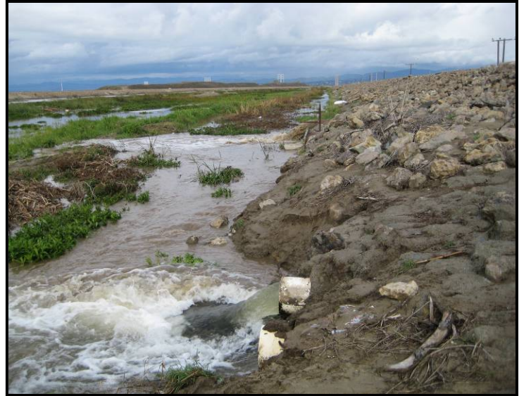
View of discharge (looking upstream on Calleguas Creek)
