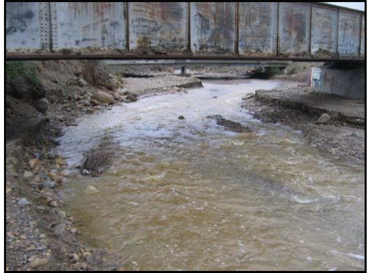
View downstream from site of RR bridge
