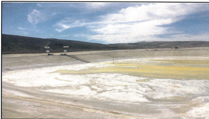
Final waste brine drying in lined surface impoundments. The surface impoundment are constructed to Title 27 requirements and regulated under waste discharge requirements.
